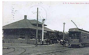
DUR Station in Orion
